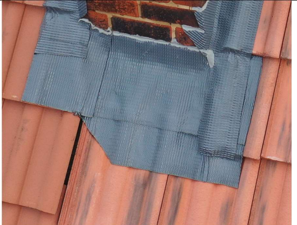
Flashing – messy detail on the front pitch.
