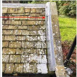
extremely weathered and cracked mortar fillet
