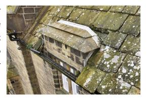
Overall, the rainwater goods appear to be in reasonable condition, however routine maintenance is due. You should budget in the first instance for adapting the circular down pipe arrangement in photo 0438 and clearing through those that are congested. The internal areas below the valley gutters should be monitored for water ingress, the GRP coatings will need replacement at some point.
